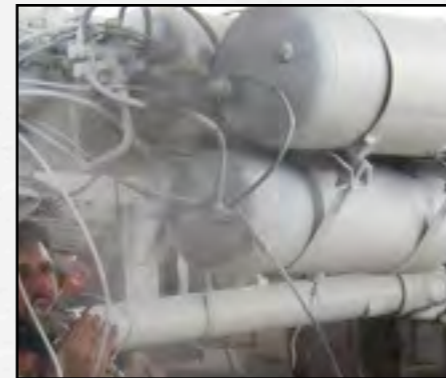
Corrosion Prevention & Insulation U.A.E.
