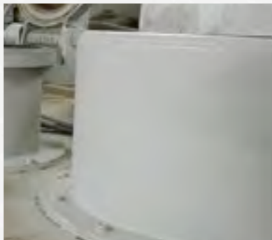
Example of a smoothed and painted EPX surface.
