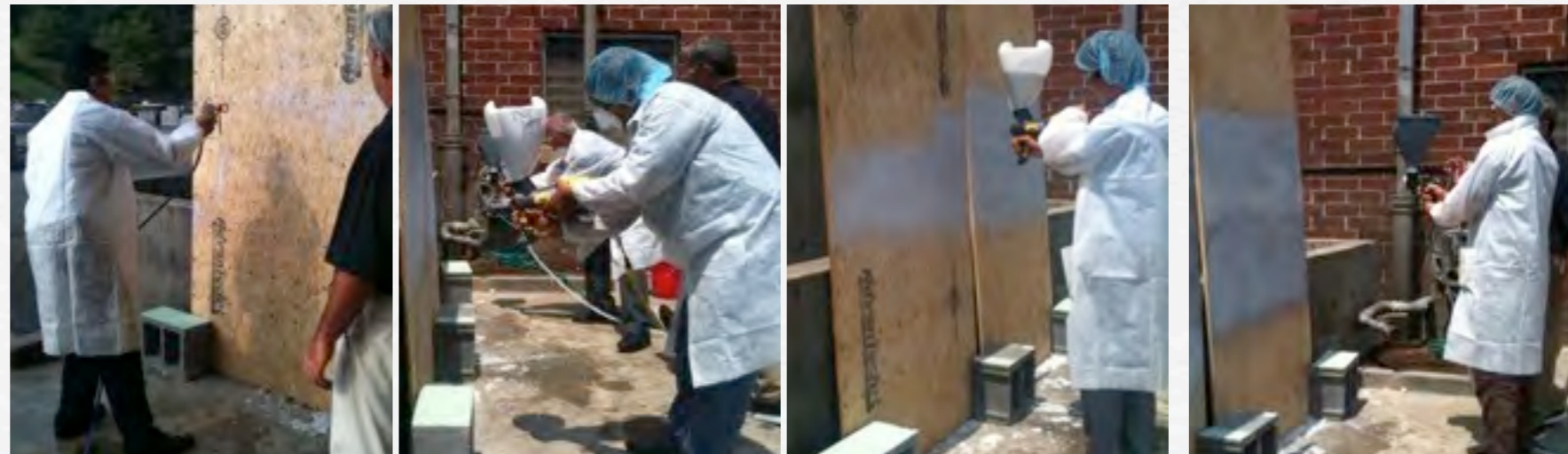
Practice with Texture Sprayer for Nansulate® EPX
