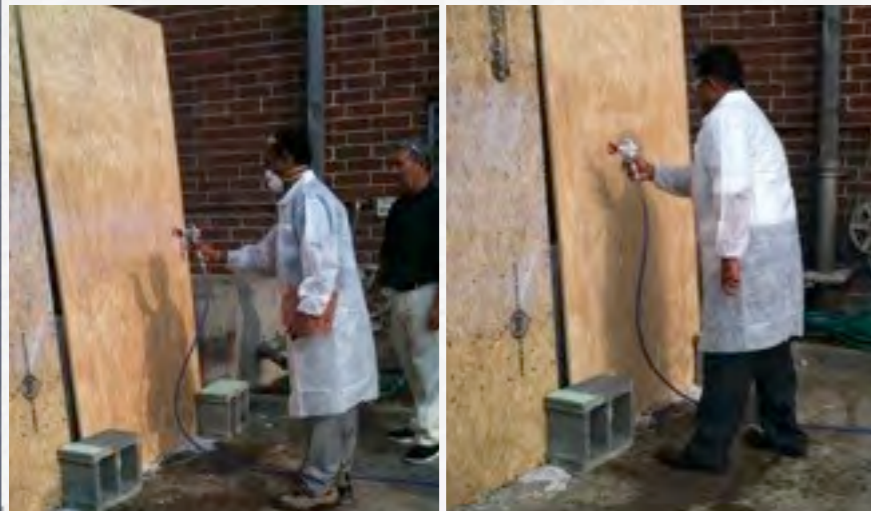
Practice with Airless Paint Sprayer for Nansulate® Translucent
