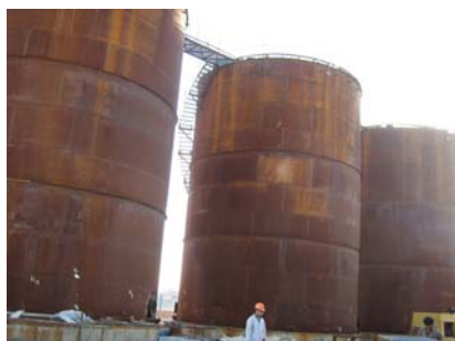
Large tanks holding methanol before application of Nansulate®
