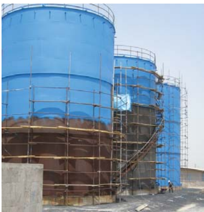
Nansulate® stopped vaporization of methanol with effective insulation properties, and offered corrosion protection and resistance to moisture penetration
