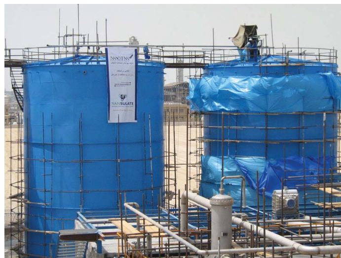
The completed, Nansulate® coated tanks provided the protection that the customer was looking for and stopped the vaporization issue while offering protection from corrosion and moisture.
