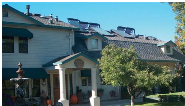
Solar array on house includes the combination of evacuated tube panels and flat plate panels. Nansulate® improved the overall performance of the solar system by reducing heat transfer from the flat plate panels.
