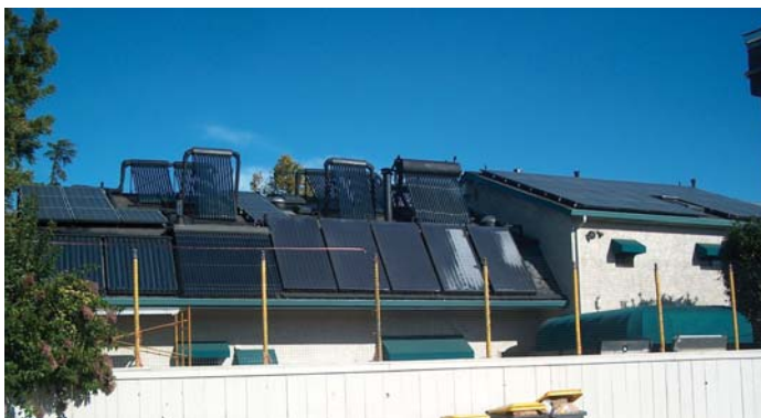
Solar array on house includes the combination of evacuated tube panels and flat plate panels. Nansulate® improved the overall performance of the solar system by reducing heat transfer from the flat plate panels.
