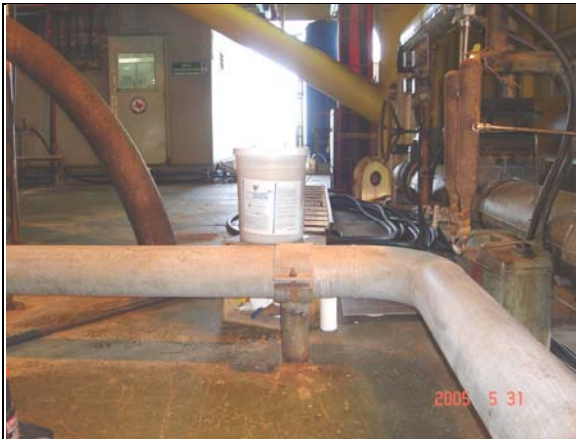
View of the final section before the work
