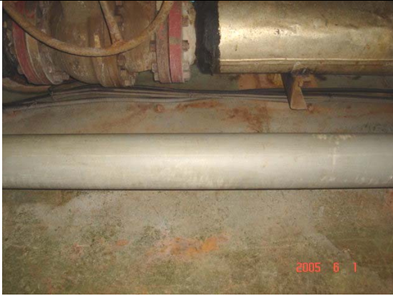
Final aspect without primer. Middle section
