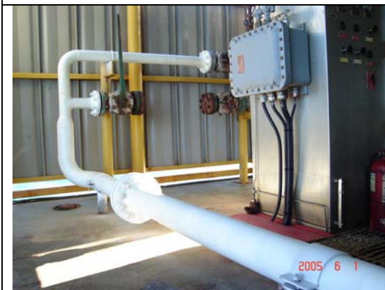
First section. Work done
