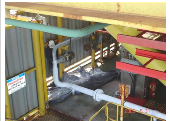
First section during work.
