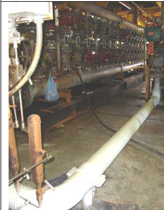
Last trace of the pipeline before pumping.
