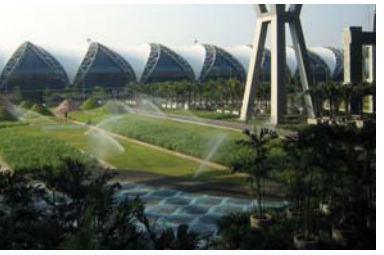
The panels are used as roof and soffit claddings for the terminals aerobridges
