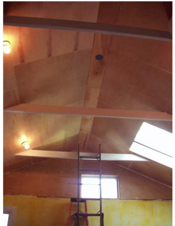
Over wood cathedral ceiling
