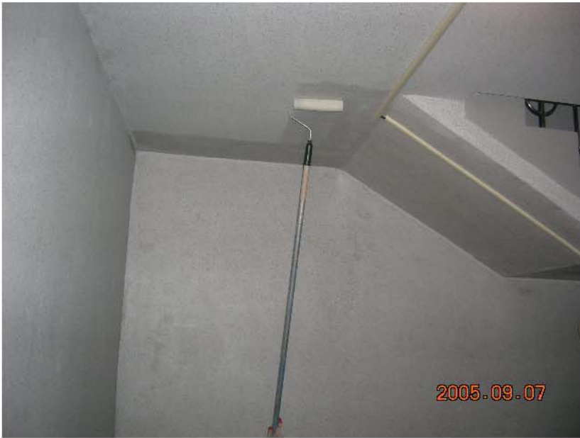
Over pre-painted wall & ceiling
