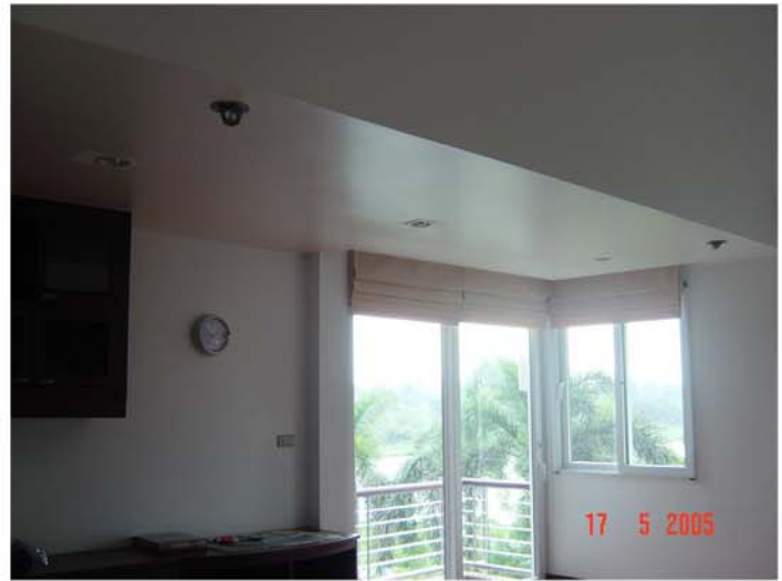
Over pre-painted wall & ceiling
